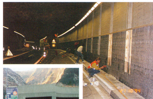
LIDA® NET installed in the San Gottardo tunnel Switzerland
