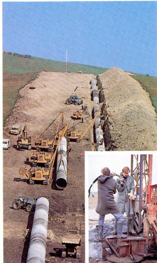
LIDA® anodes are installed in conventional or deep groundbeds to protect transmission and distribution lines.
